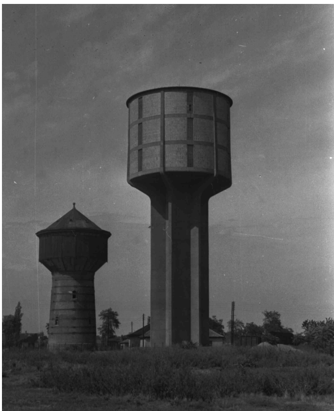
Fig. 17. Old and new water towers together at the Szolnok Railway Station, 1952. Courtesy of MÁV Archives.
