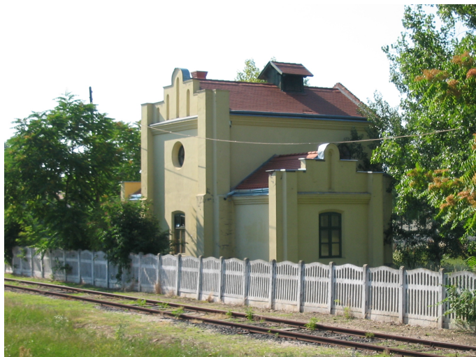
Fig. 1. The water house of the Ó-Szolnok station, built ca. 1850 was renovated for the 150 th anniversary of the inauguration of the Pest-Szolnok line.
