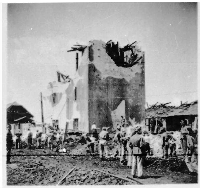
Fig. 16. Bomb hit older station water tower in the summer of 1944, (b. ca. 1850). Courtesy of the Municipal Archives in Szolnok.
