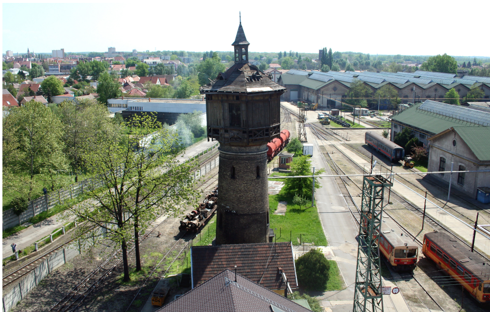
Fig. 13. Service water tower on the territory of the Vehicle Repair Enterprise in Szolnok, b. 1900.
